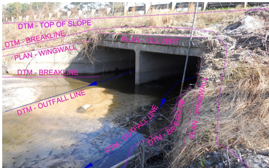
Figure 63 Culvert Survey Example
