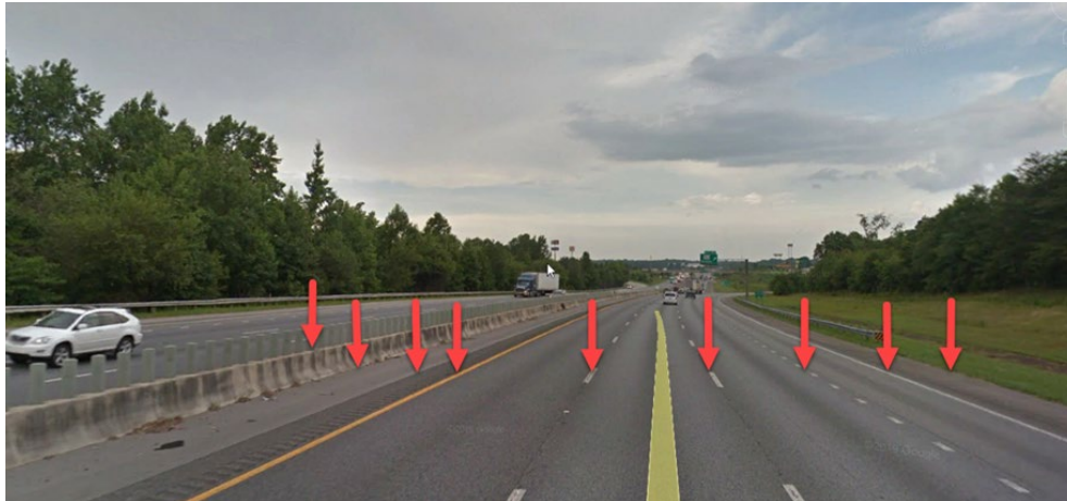
Figure 9 Interstate 3D Breakline Features
