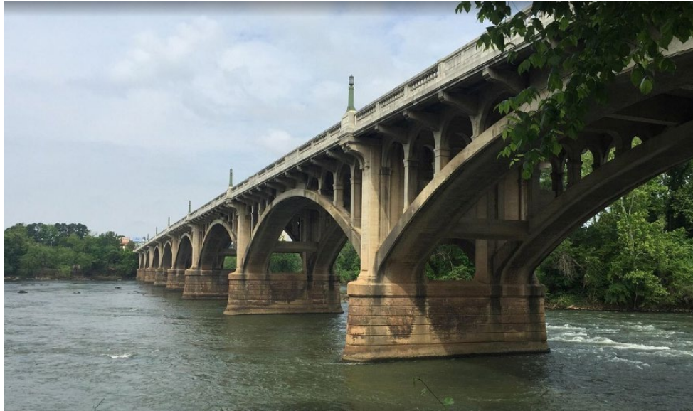
Figure 39 Example of Gervais Street bridge over Congaree River
