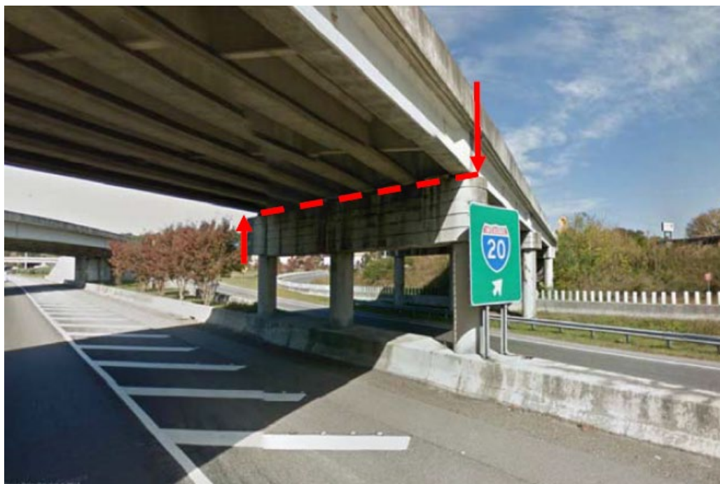
Figure 51 Bridge Bent Cap (bearing seat) Survey Locations
