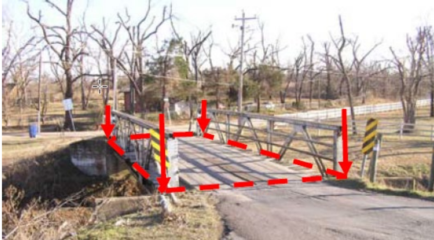
Figure 53 Wooden Bridge Deck Survey Locations
