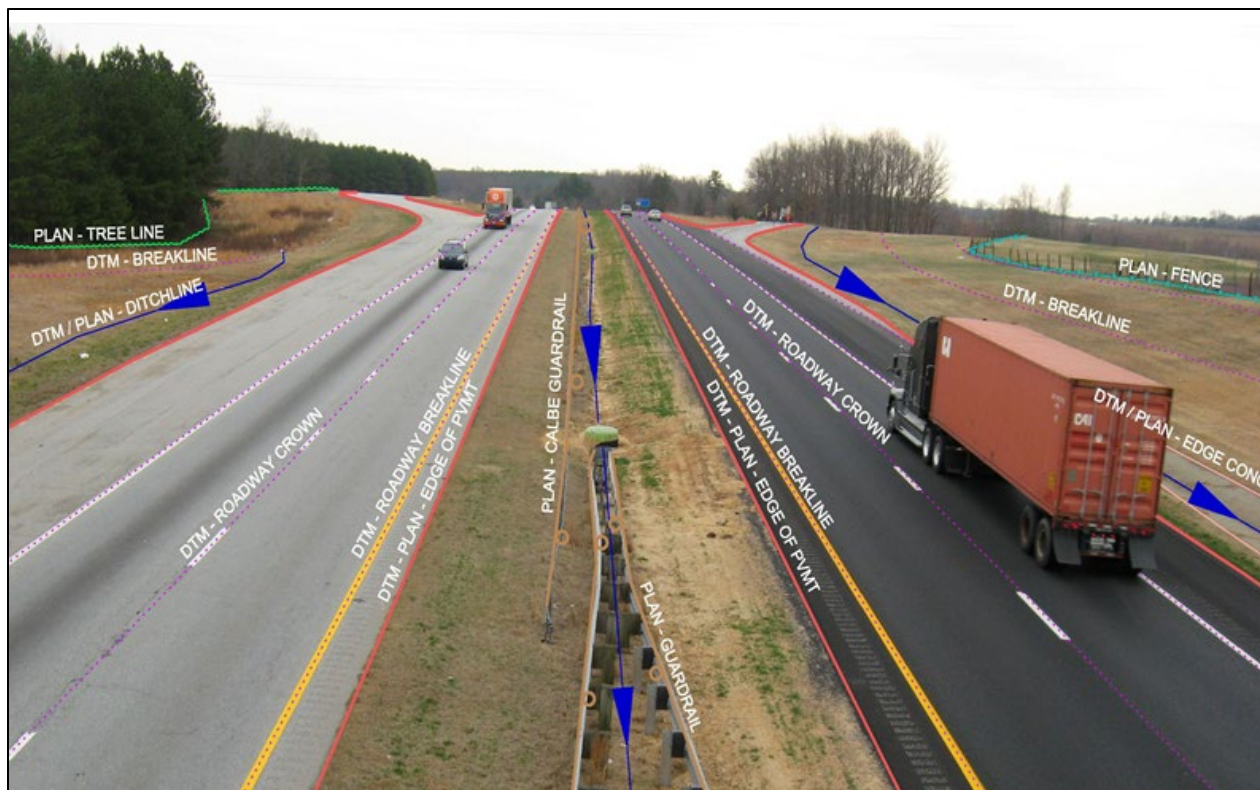
Figure 34 Highway Survey Example
