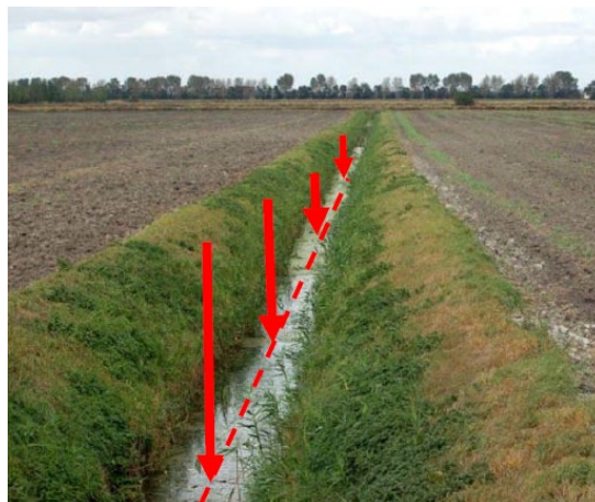
Figure 36 Example of Outfall Ditch Flowline
